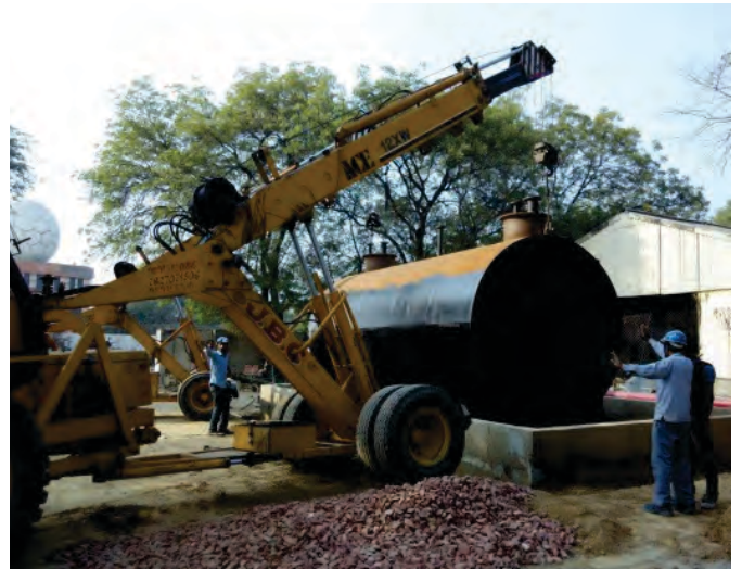
Modernization Project : Installation of 45 KL tank in Fuel Farm
